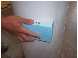
Screw in place. Tape and mud recessed seam. Sand seam smooth with radiused sanding block (included). Paint & finish
