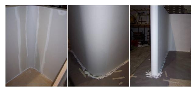
Screw in place like drywall. Tape & Mud like drywall. Finish & paint like drywall
