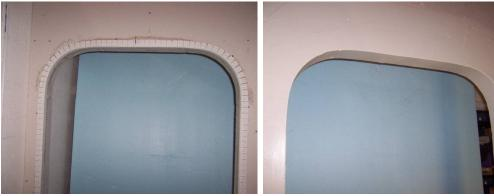
No extra framing. No need to bend drywall. Screw corners in place. Add flat strips of drywall around the jam. Install facesheet over opening, screwing into doorframe and blocking. Roto-zip opening. Trim with preffered edging. Finish as normal.
